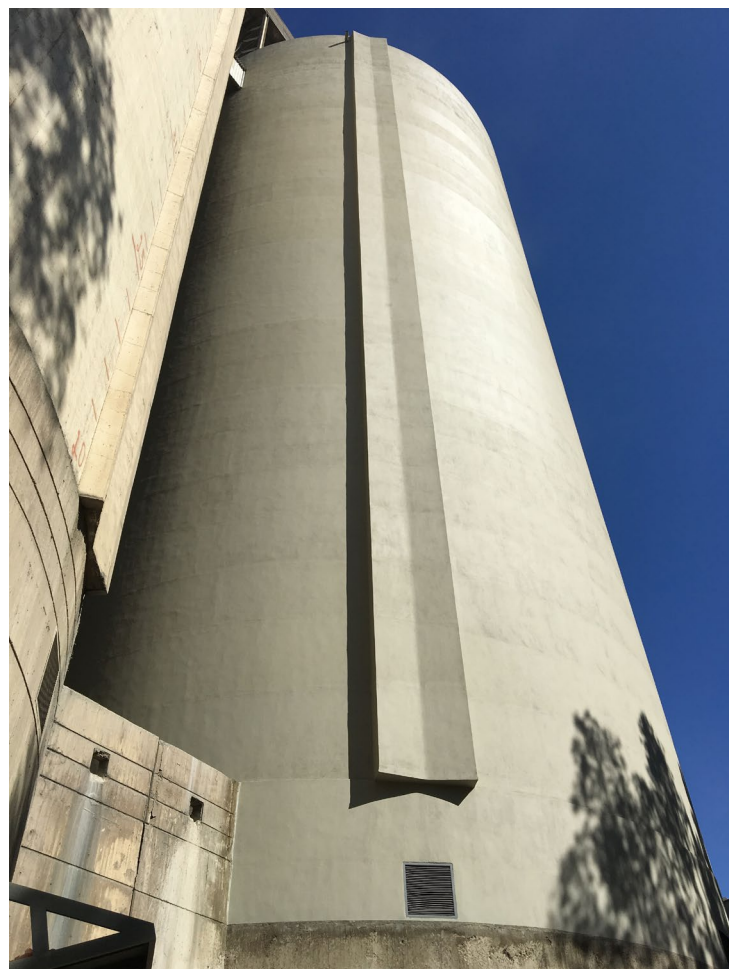
After remedial works.
