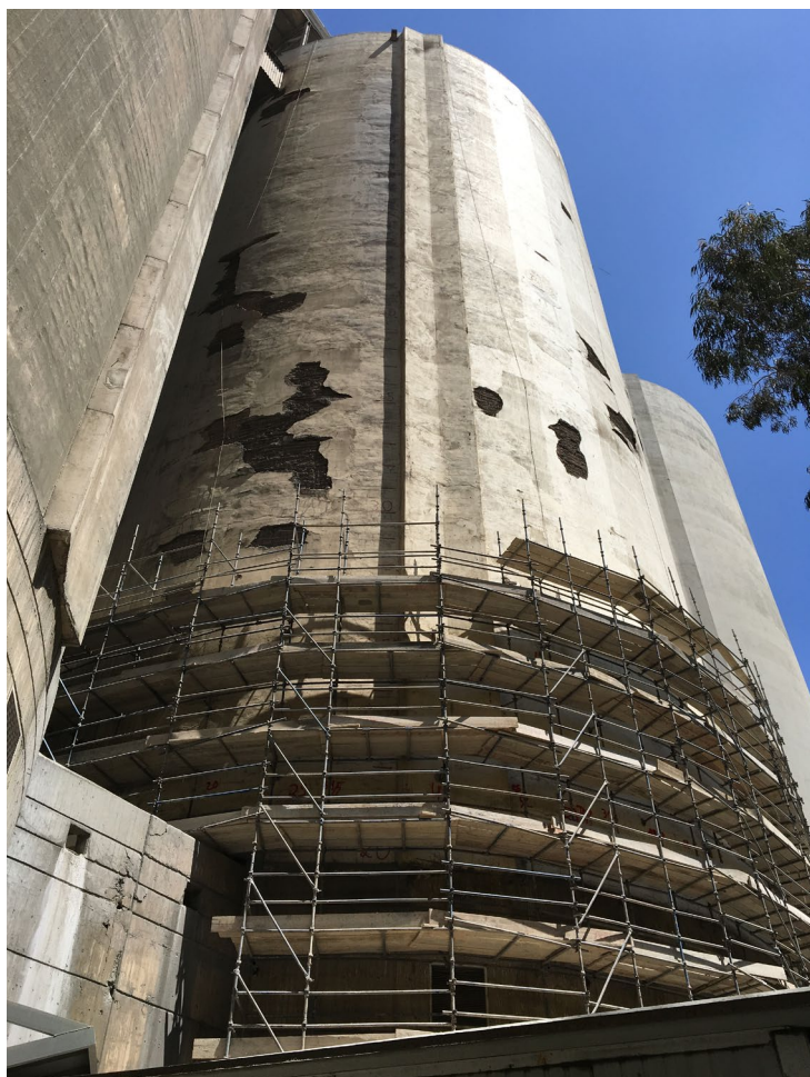
Before remedial works.
